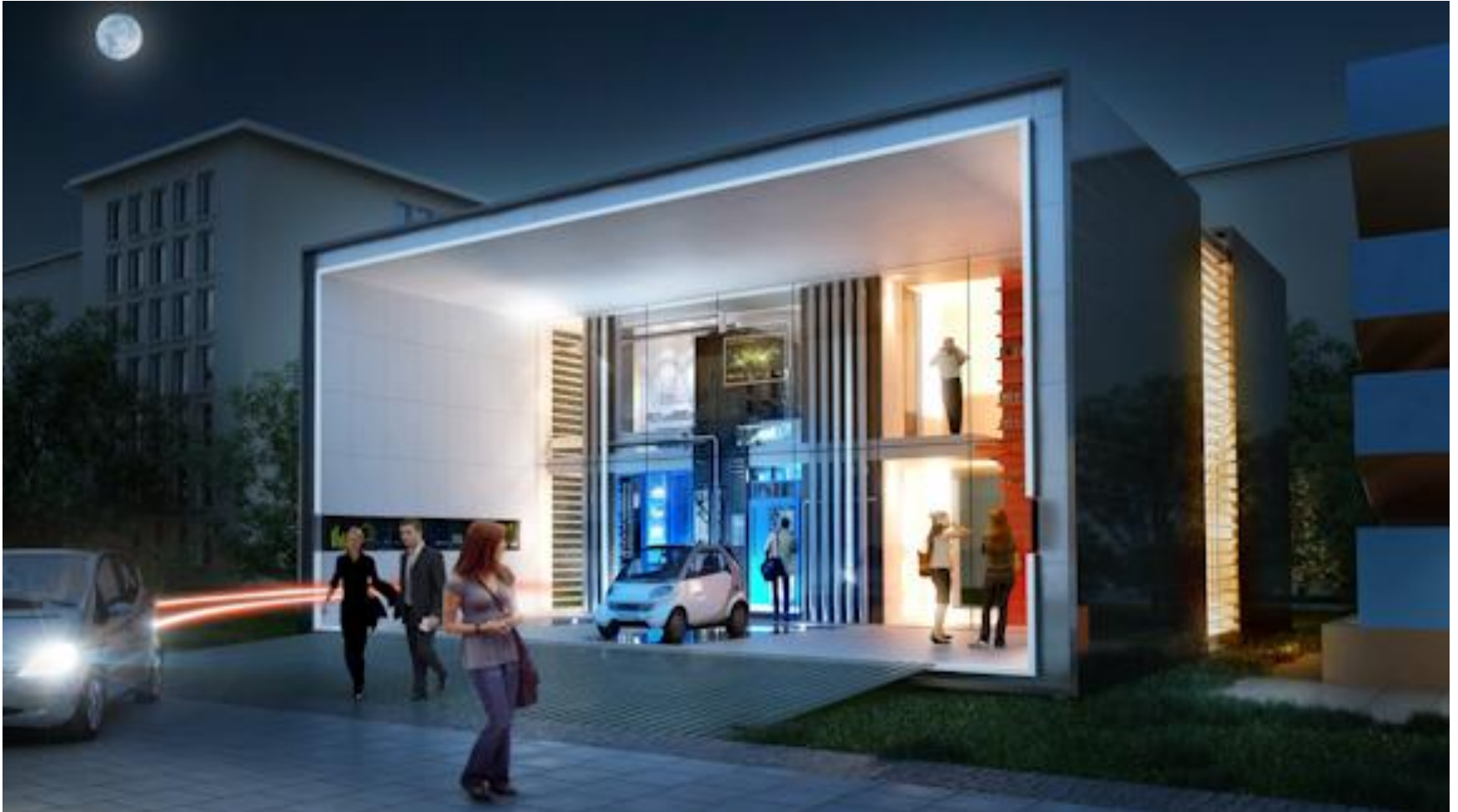
Energy plus house in Berlin (Source: Werner Sobek)
