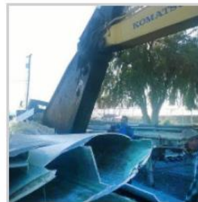
Blades are broken into pieces.
