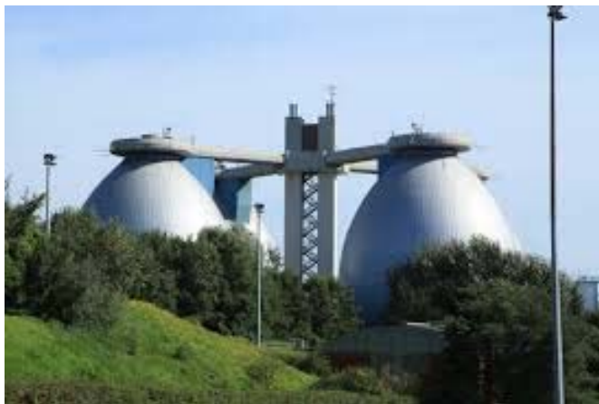
Waste and waste water treatments
